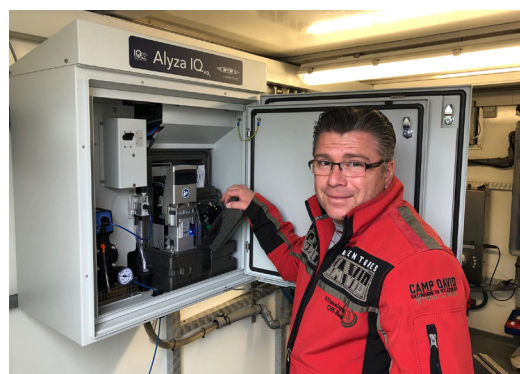
Figure 1: The Alyza IQ PO4 on the Polish plant of the city of Skarszewy (near Gdansk).
