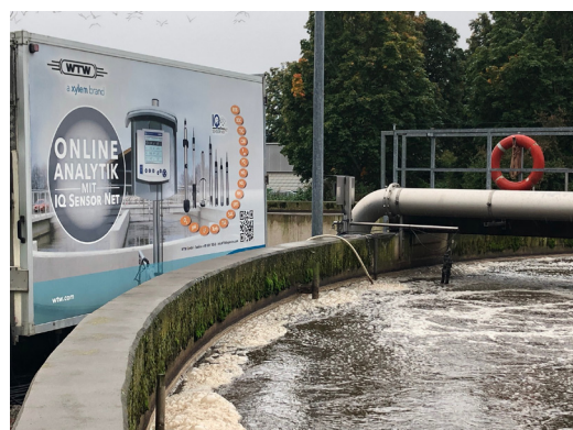
Figure 2, 3: Our sales representative Marcus Nickel and his measurement trailer at the Bückeberg sewage treatment plant
